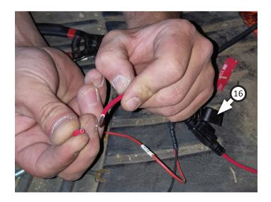
19. Insert stripped ends of fuse holder and control unit into **butt connector (18)**. Crimp connection, then apply heat to middle of butt connector to seal wires together.
